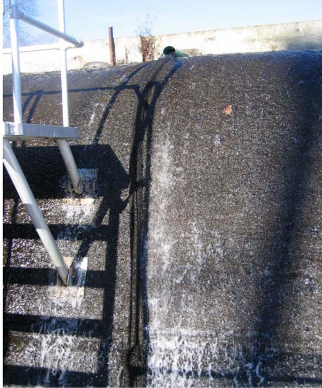
**Figure 3.** View of eel pass netting hanging over spillway on the Mianus River Dam in CT in an area of reduced flow created by the face-boards.
