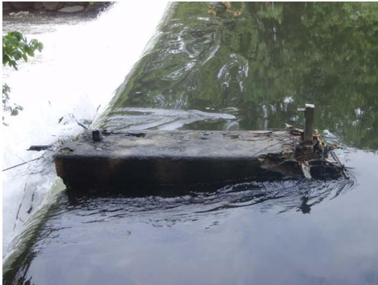
**Figure 7.** Cement structure located on the top of the 182<sup>nd</sup> St Dam viewed from the east retaining wall. Face-boards could be attached to the upstream façade of the structure to reduce flow and prevent juvenile eels that climb the net from being carried back over the spillway.
