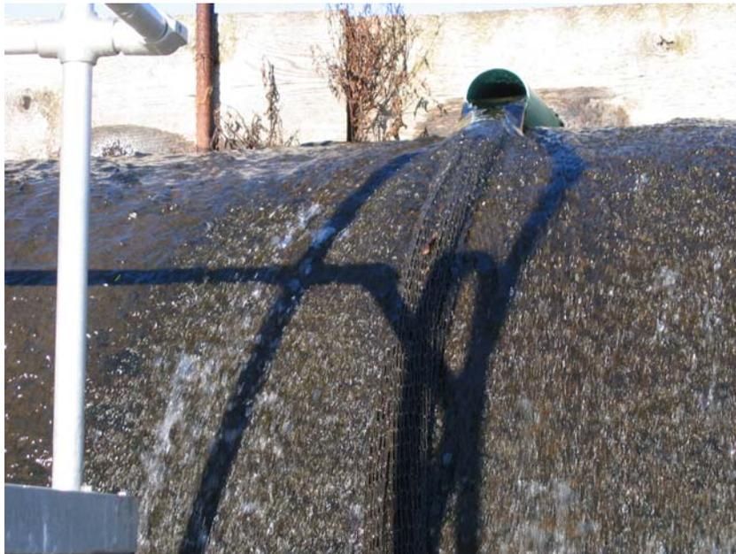
**Figure 2.** Close-up view of the trawl netting entering the PVC tubing on the Mianus River Dam in CT.
